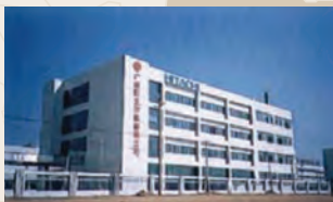
Hitachi Air Conditioning & Refrigerating, Китай
